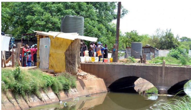
Informal settlements and pit latrines on the banks of the Crocodile (West) Irrigation Scheme below Hartbeespoort Dam.
