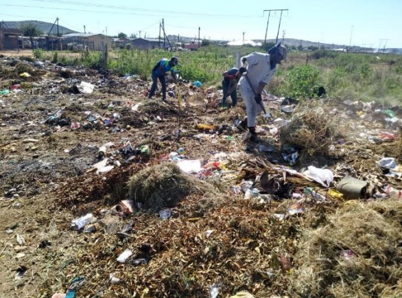
Site before intervention
